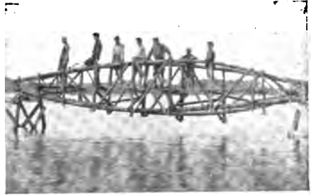
BOYS BUILDING A BRIDGE: BOW-STRING SPAN IN POSITION
